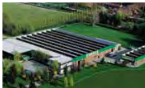
Our current Vortice Headquarters have been located in Tribiano (Milan) since 1972.
